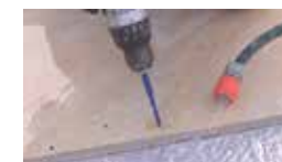
TD850V Pilot / guide hole drilling
